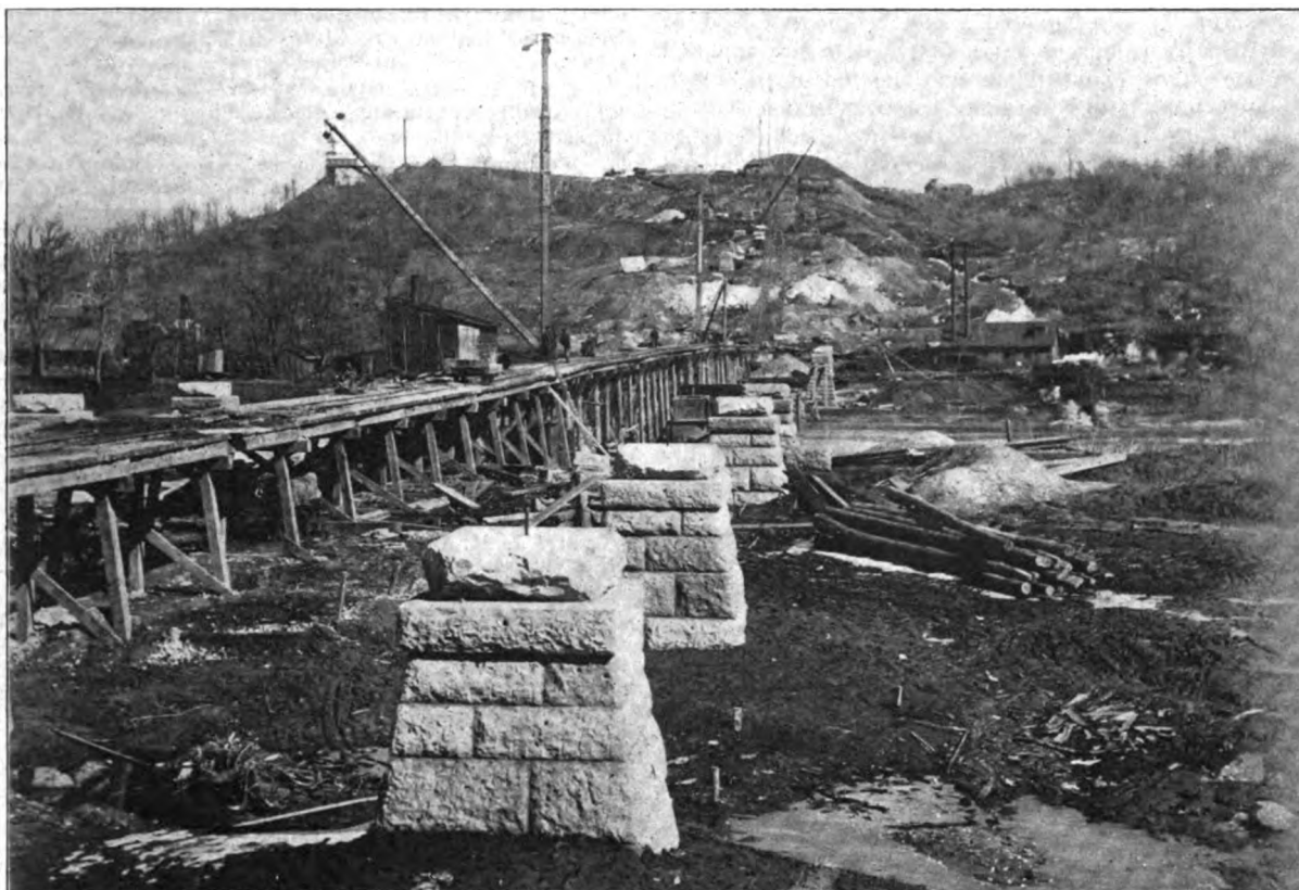
VIADUCT AT BOONE, IOWA, CHICAGO & NORTHWESTERN RAILWAY—VIEW SHOWING STONE PIERS FOR TOWER FOUNDATIONS. From photograph taken March 10, 1900.
