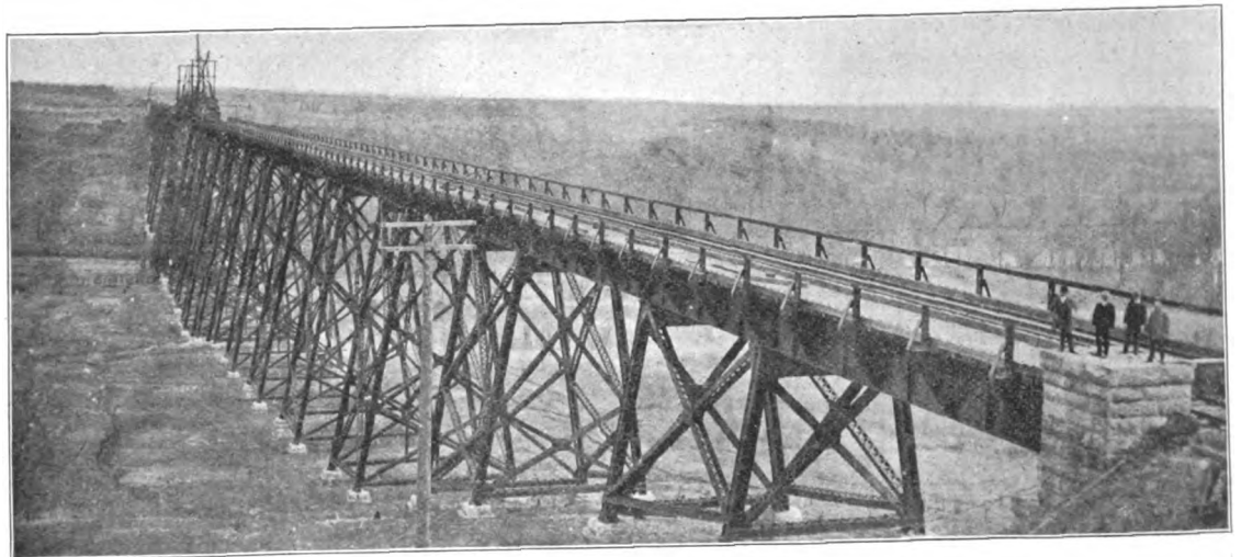
FIG. 4, BOONE VIADUCT, CHICAGO & NORTHWESTERN RY.—COMPLETED STRUCTURE.
