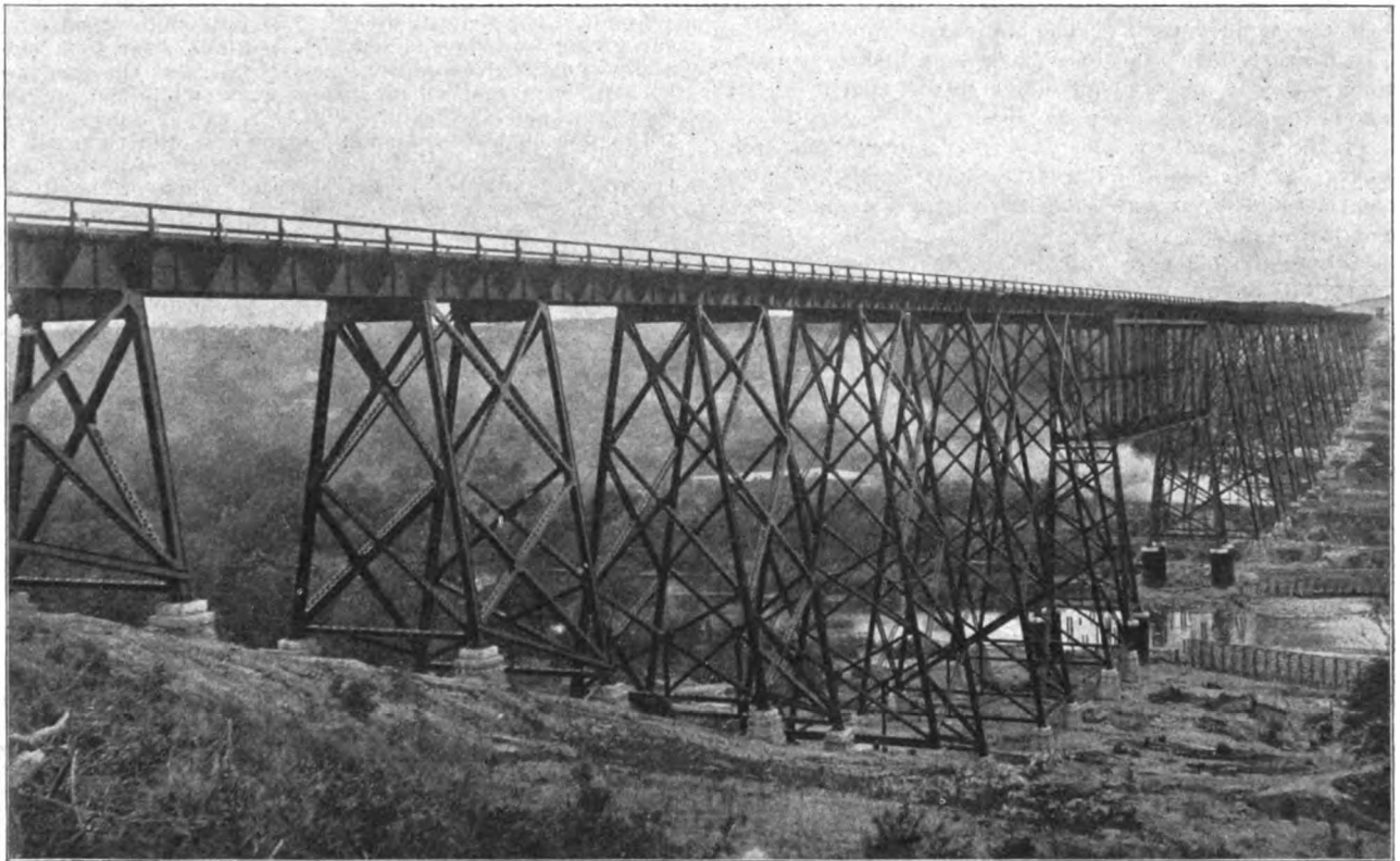
VIADUCT AT BOONE, IOWA, CHICAGO & NORTHWESTERN RAILWAY—VIEW OF WORK AFTER COMPLETION.
